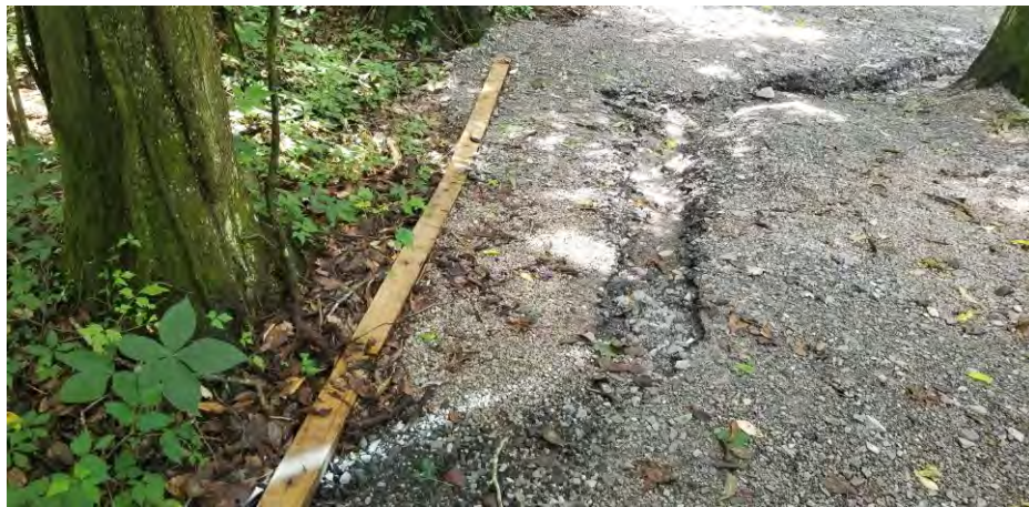
Figure 62. Erosion of a BREC trail following a heavy rain event (Source: BREC Staff).
