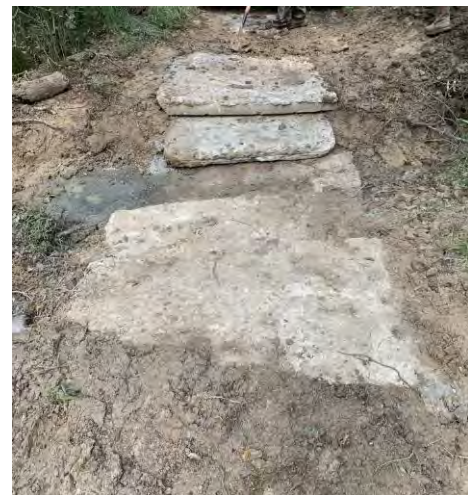
Figure 64. Reinforced pathway made of steps where trail crosses a small stream channel at BREC's Frenchtown Conservation Area. (Source: BREC staff)
