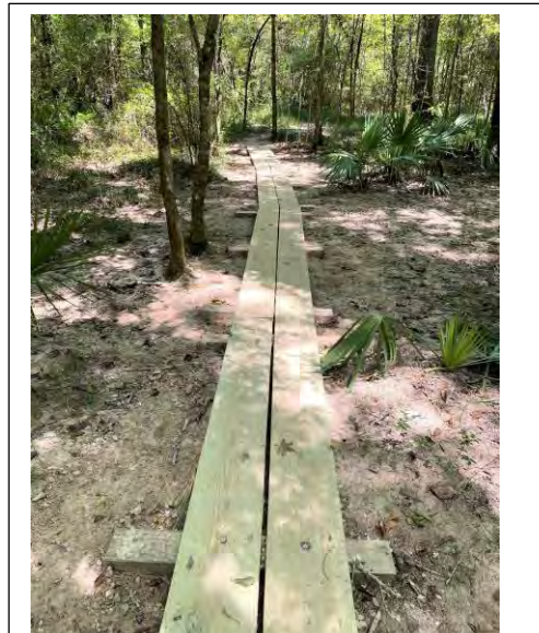
Figure 57. Bog bridge for hiking pedestrians at Kendalwood Conservation Area (Source: BREC Staff).
