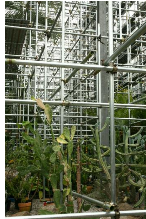
Scaffolding in the Tsukuba Botanic Garden greenhouse while repairing earthquake damage
