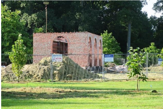
Photo 15: Construction of the Artois Pavilion, September 2019
