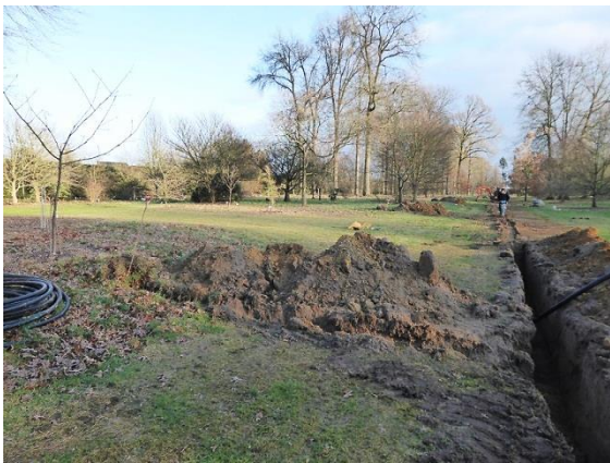
Photo 3: Irrigation works in the Werner Wood
