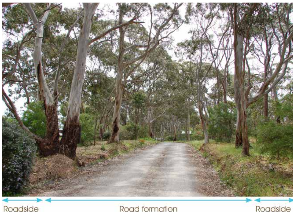
Figure 1. Road reserve showing road formation and roadside. See also diagram on page 69.
