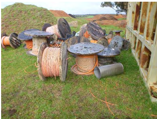
Plate 5-8 Dumping of materials with the Project Site to the south of the retention dam.
