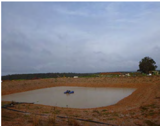
Plate 5-6 Retention dam with area leased by Plantation Energy on the northern boundary.
