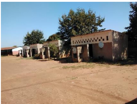
4th of October Primary School Sanitaries, Nhamatsane
