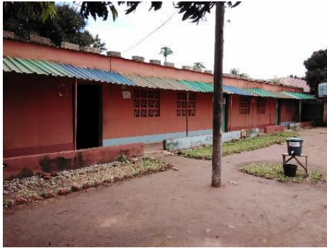
AKA Power Primary School, Bairro 5
