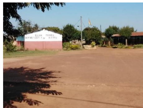
4th of October Primary School classroom block, Nhamatsane
