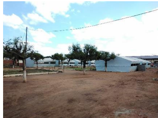
Temporary rooms at Fepom Complete Primary School,, Bairro 5
