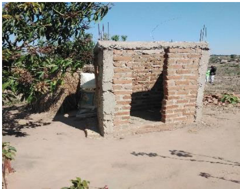
House under construction made of burnt clay blocks, Vila Nova
