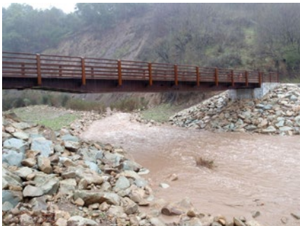
Lion Creek Bridge Improves Fish Passage. In 2010, a “fair weather crossing” on Lion Creek, a major tributary of San Antonio Creek, was replaced with this bridge, which improved steelhead access to over nine miles of upstream habitat. Photo courtesy of South Coast Habitat Restoration
