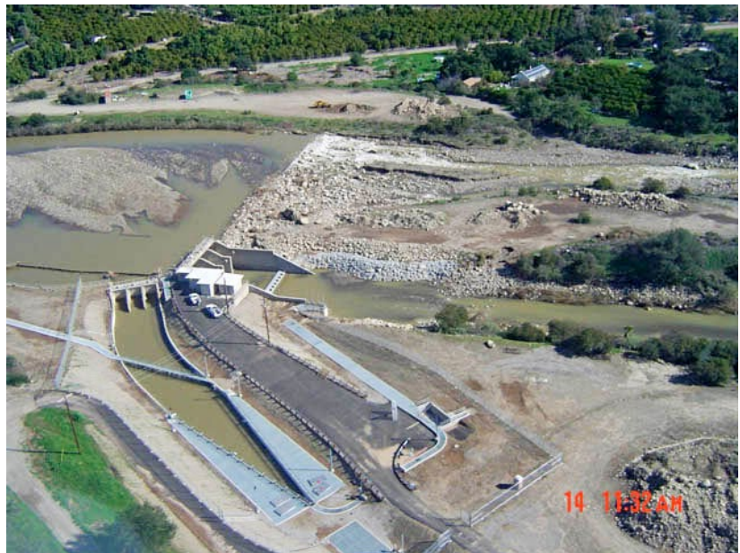
Robles Diversion and Fish Passage Facility
