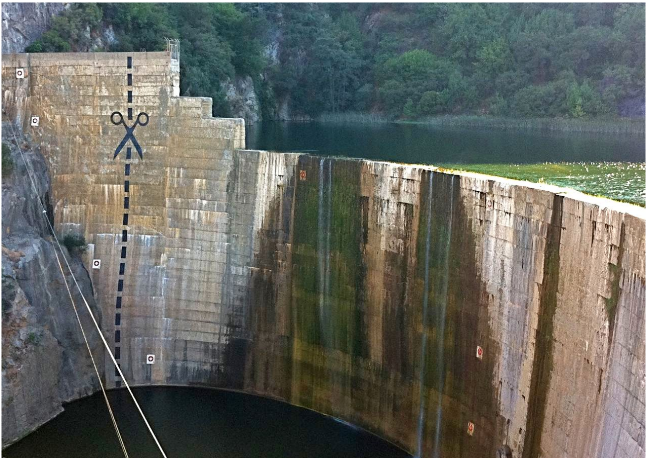
Matilija Dam Notches. The top of the dam was notched in 1965 and again in 1978 to address safety concerns, including strain on the dam from water stored behind the dam and deteriorating concrete. The original dam height was 198 feet and is now 168 feet (USACE 2004). In 2011, someone painted a huge pair of scissors and a long dotted line on the face of the dam.
