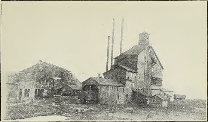
FIG. 1.—View of Iowa Coal-Washing plant, Lakonta.
