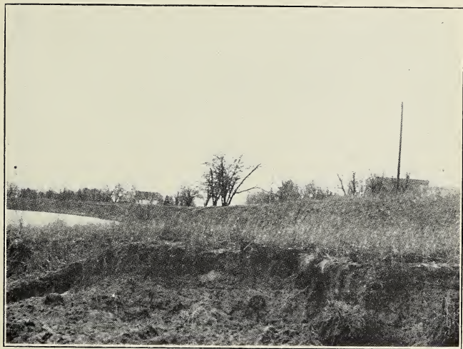
FIG. 2.—View of a portion of the old excavation east of the track at Avon, Iowa. Here the water is but three to four feet deep. The stratification of the sand and gravel is very evident in the foreground.
