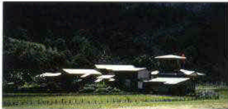
Airport buildings, Ba'Keklen
