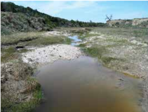
Photo 5. Recent channel widening is evident from a combination of sparsely vegetated streambanks, slump blocks, cutbanks along straight channel segments, and a high width/depth ratio along much of the reach.
