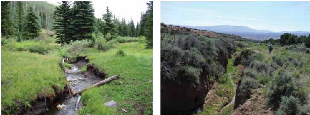
Figure 9. The photo on the left shows an example of a stream that can no longer access its floodplain. Item 1 would be answered “no.” The photo on the right shows an example of a channel that has incised but has begun to rebuild a new floodplain in the inset channel. Item 1 would be answered “yes” for this type of situation.
