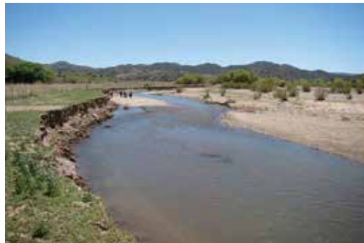
Figure 32. Evidence of bank erosion in an unstable channel could include slumps, sloughs, fractures, or slides. On this stream, the banks have eroded along long (several hundred meter), continuous spans. Eroded bank material is added to the channel and increases sediment load.
