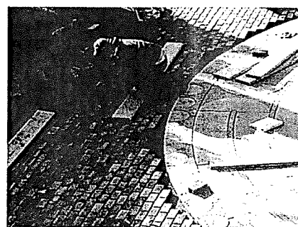
The brick surround is getting finished
