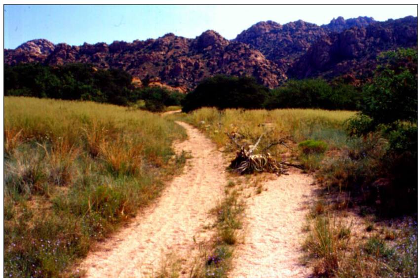
Figure 3.6B Slavin Gulch Road after closure, March 2000 (Right track shows areas with, versus without revegetation.)
