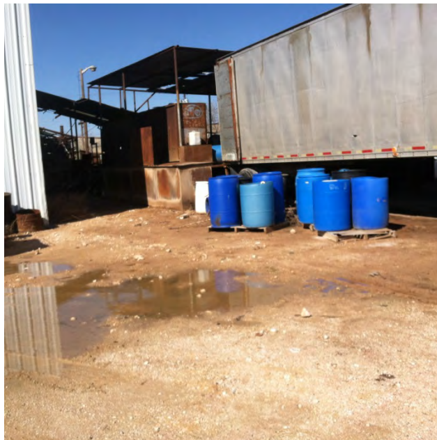
Photo 16: Drums, tractor-trailer, pooled water, and the condition of the structures near the loading dock. Facing west-northwest. Photographer: Kristen Kochelek
