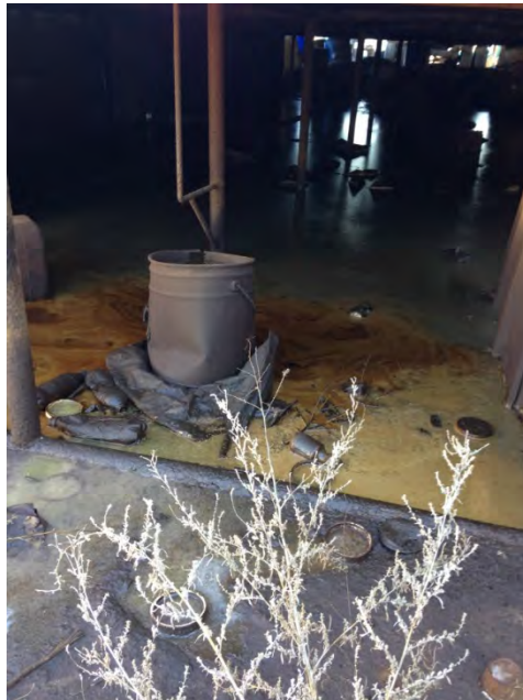
Photo 5: Frozen liquid underneath loading dock on ground surface. Facing southeast. Photographer: Katie Delbecq
