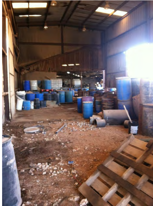
Photo 11: Inside of the drum unloading area and the processing area showing stained soil and overturned buckets along with the condition of the structure. Facing west-northwest. Photographer: Kristen Kochelek
