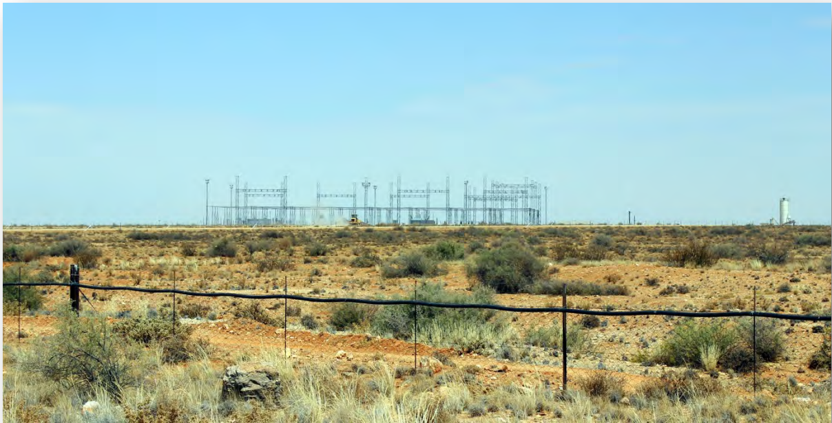
Figure 8.5: Nieuwehoop Substation currently under construction (Photo site SCA010)
