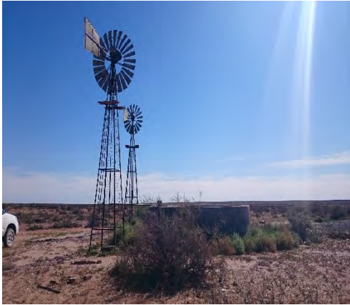
BH1 - wind pump
