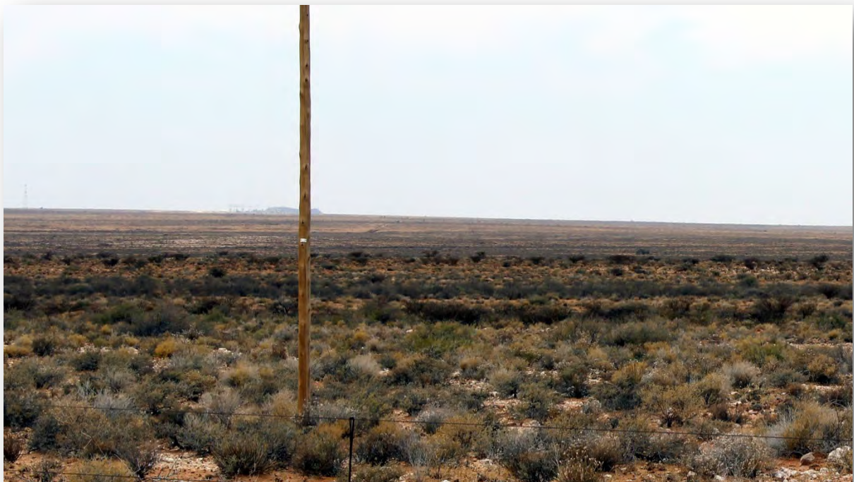
Figure 8.4: View from photo site SCA014 eastwards. The tower at Rugseer Siding is visible on the left and the new substation more towards the centre.
