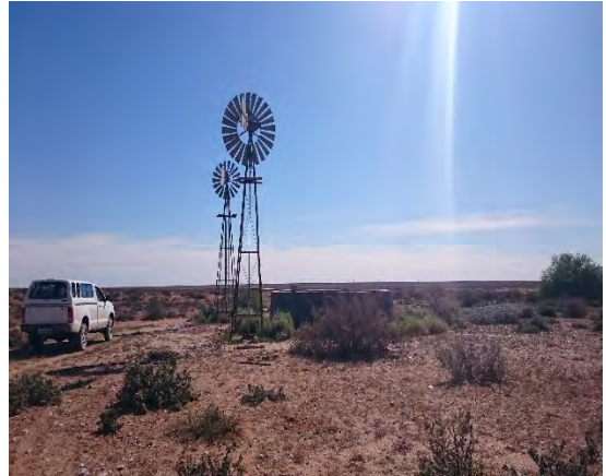
BH2 - wind pump
