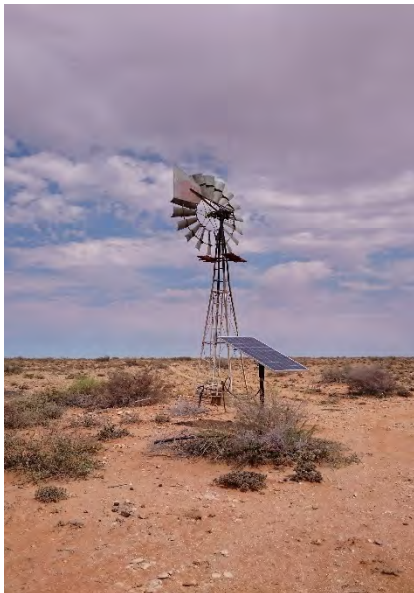
BH5 - wind pump
