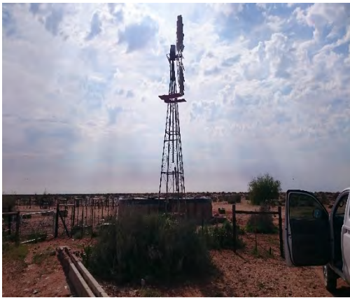
BH3 - wind pump
