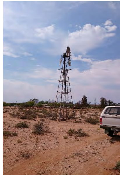
BH6 - wind pump
