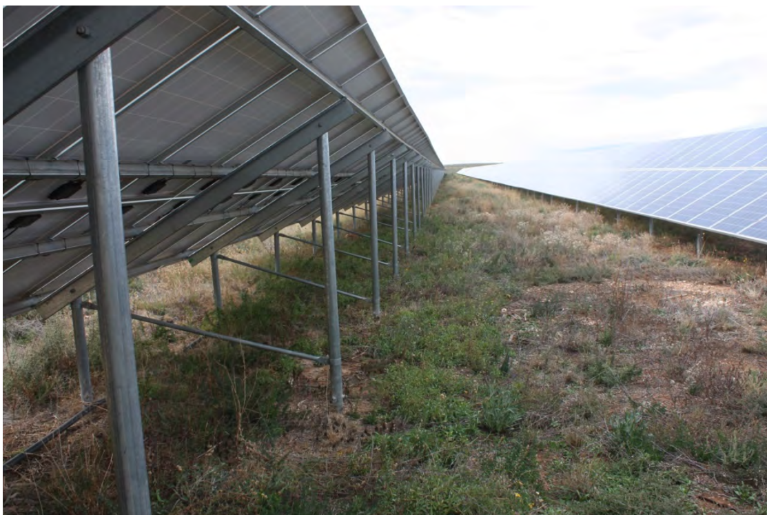
Figure 7.9: Image of solar arrays indicating the limited influence that such structures generally have on the flow of surface waters within a solar facility.
