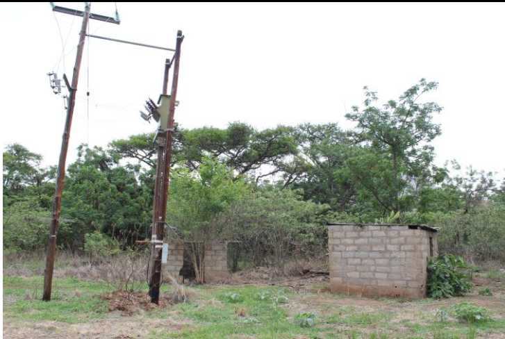
Figure 9: Redundant farm infrastructure is found on the project sections B and C.
