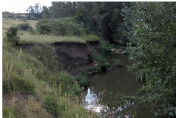
Bank collapse and scouring
