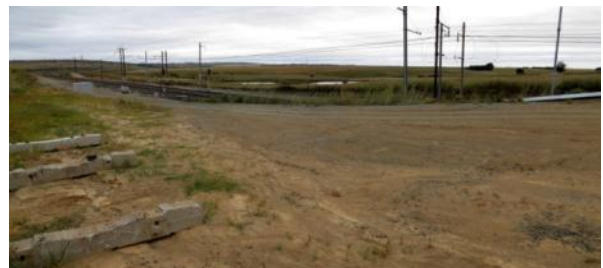
Railway infrastructure in the extensive seep in the southern portion of the site
