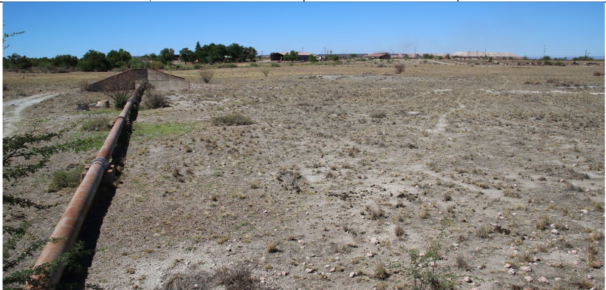
Figure A1: A view of the existing pipeline through Kathu pan.
