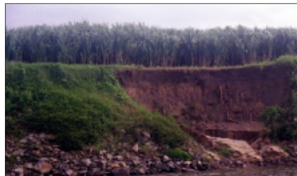
Erosion Problem in the lower Barron (Photo: Helen Adams)
