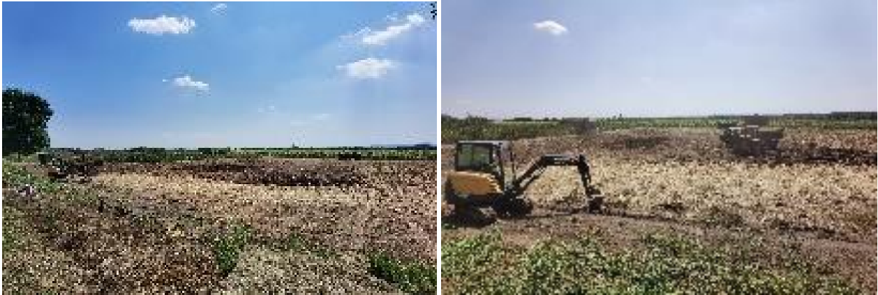
Figure 13. Restoration in process
