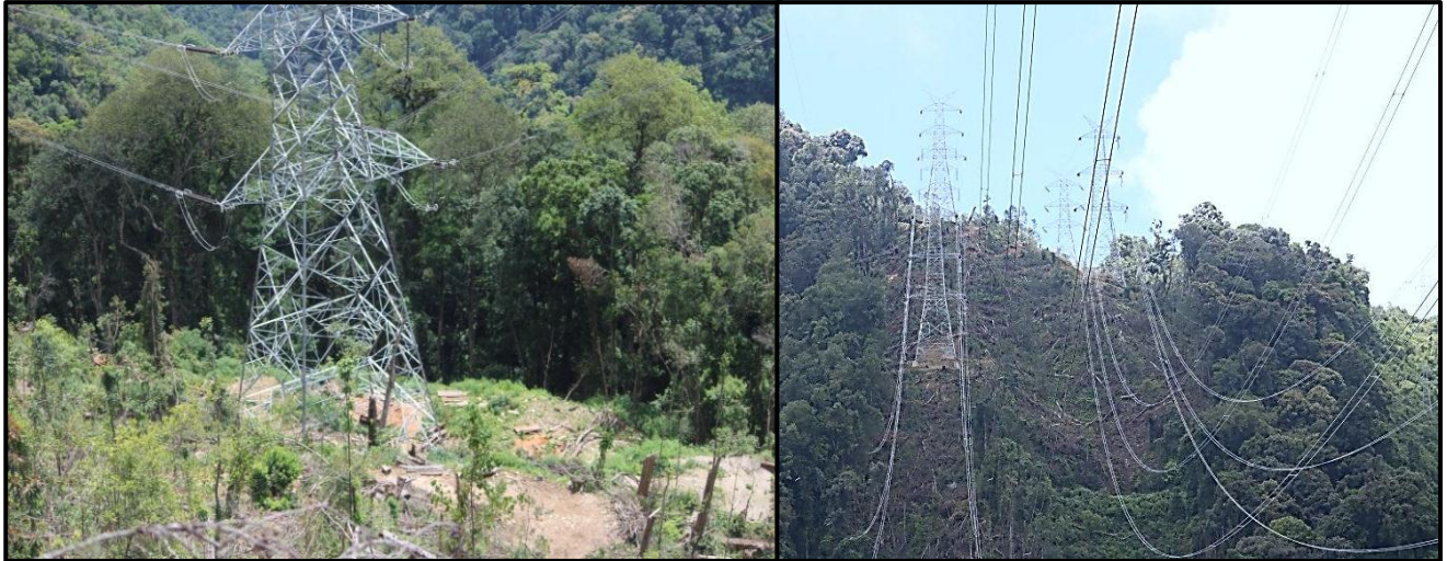
Figure 28: The high power transmission lines constructed in the habitat of RNH.
