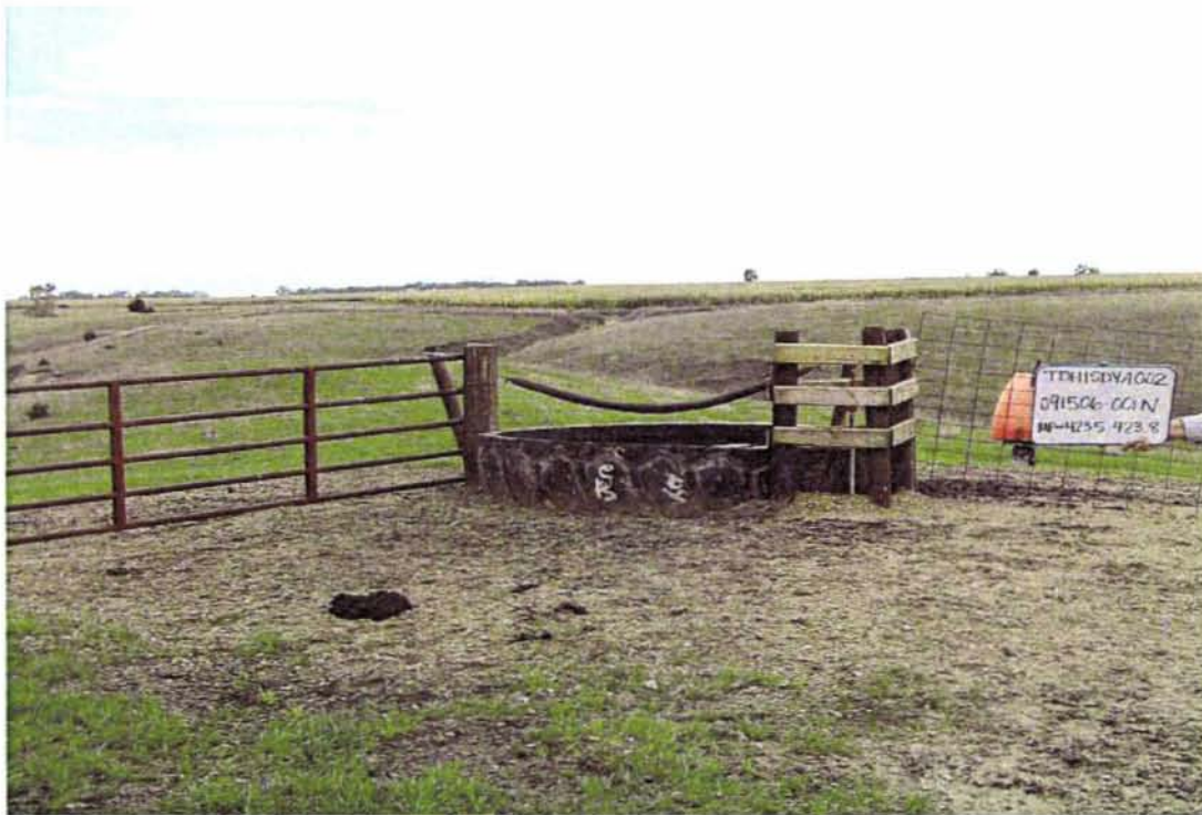
Feature TDH1SDYA002: Heavily trampled water tank at center line, along the ridge.
