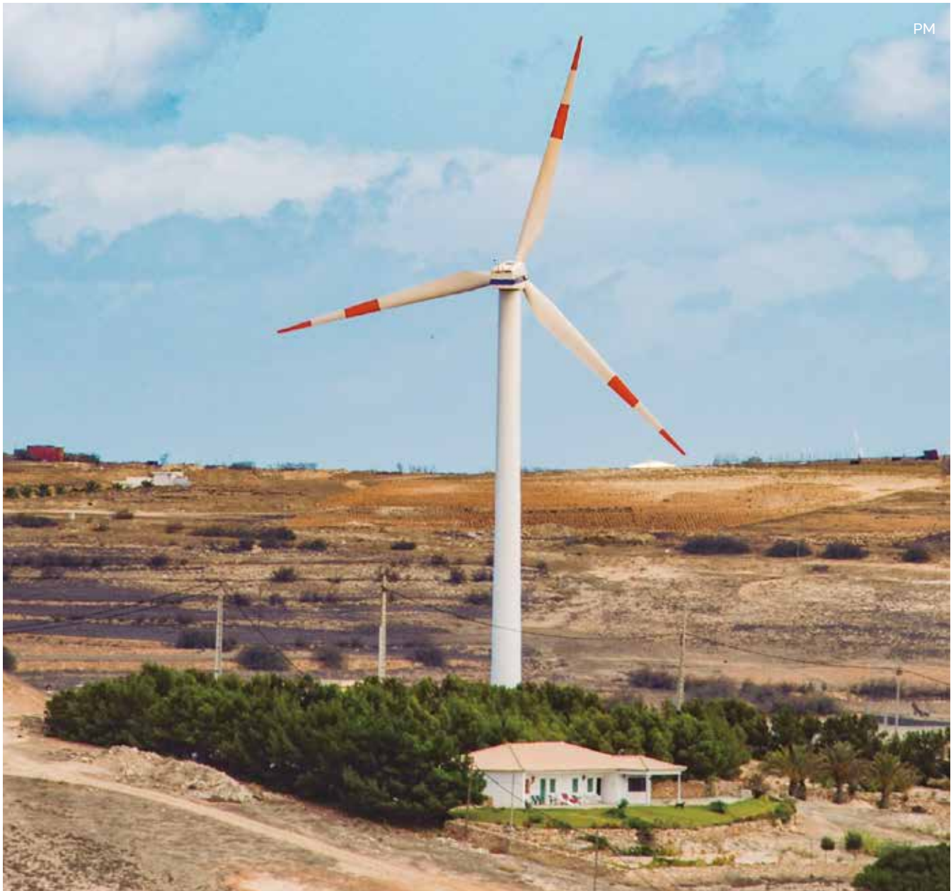
Wind generator - wind energy
