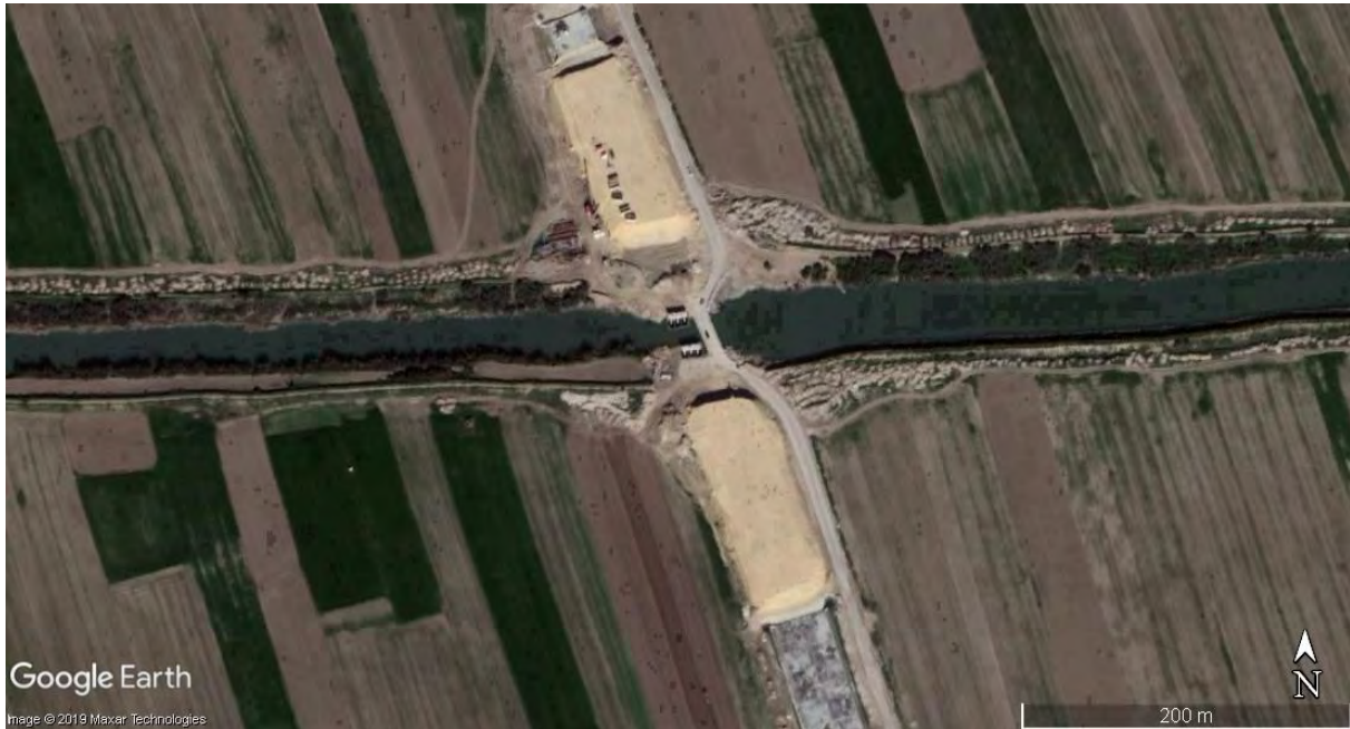
Figure 10 Construction of the crossing of the River Mejerda by the new road from Tunis to Kalaat el Andalus. Photo: Google Earth
