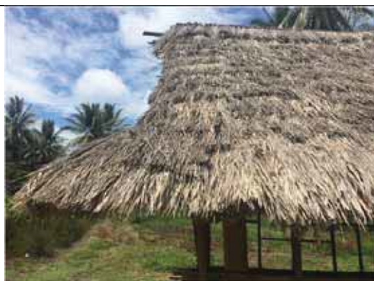
Photo 42. Roofing made out of Poatz ( Imperata cylindrica ).
