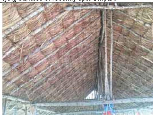
Photo 43. Internal view of Poatz ( Imperata cylindrica ) roofing.
