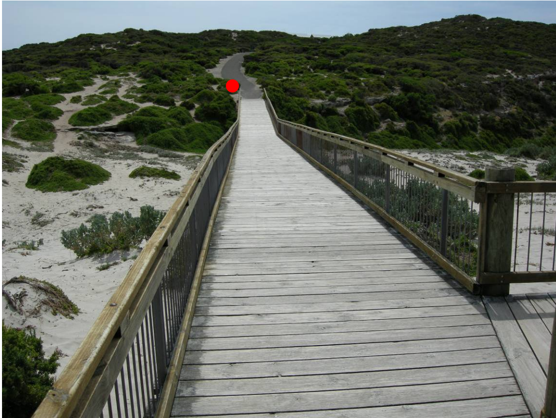
Fig. 11. View to North on the bridge between the path from the Visitor Centre and the Main Platform. The new bridge would be to the left of the picture and will extend from where the new path would end (red dot). The new bridge would be wider and approximately 700mm higher than the current bridge.
