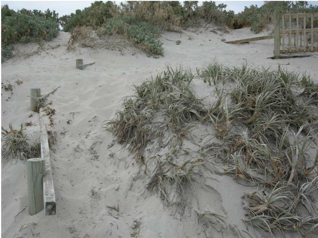
Fig. 24. View to the North taken from the beach below the platform at the end of the Don Dixon Boardwalk. The picture shows the build up of sand at the end of this platform.
