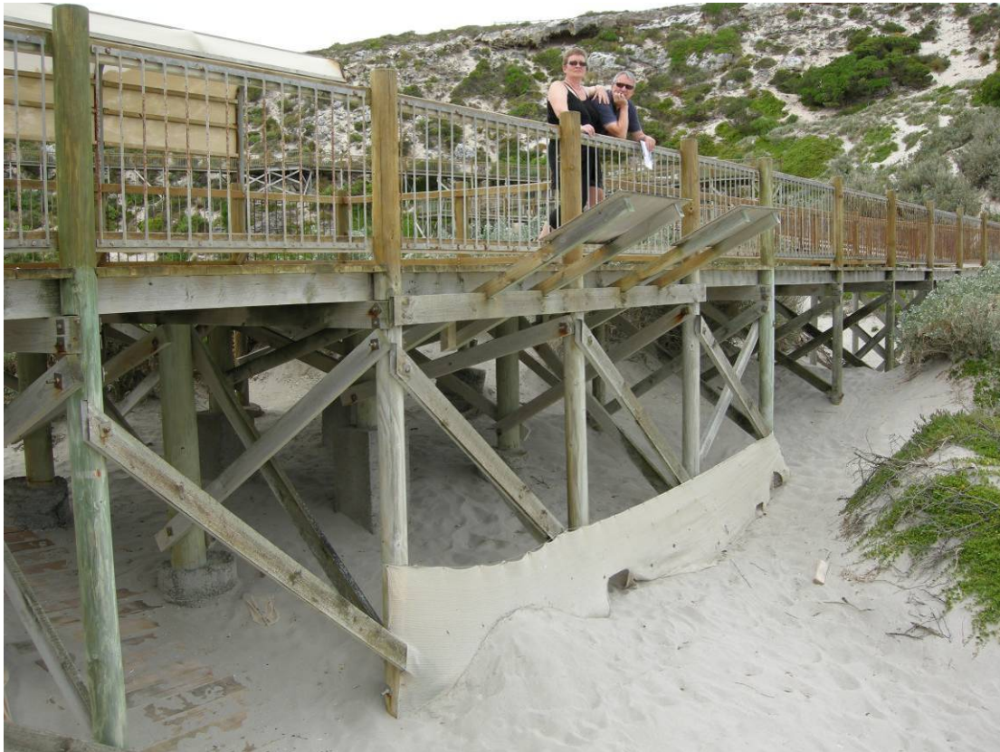
Fig. 23. View to the Northeast taken from the beach below the platform at the end of the Don Dixon Boardwalk. This platform may be widened (into the dunes, not the beach). The picture shows the exposed concrete footings and the shade cloth and duckboards that have been put in place to minimise erosion caused by wind and ASL.
