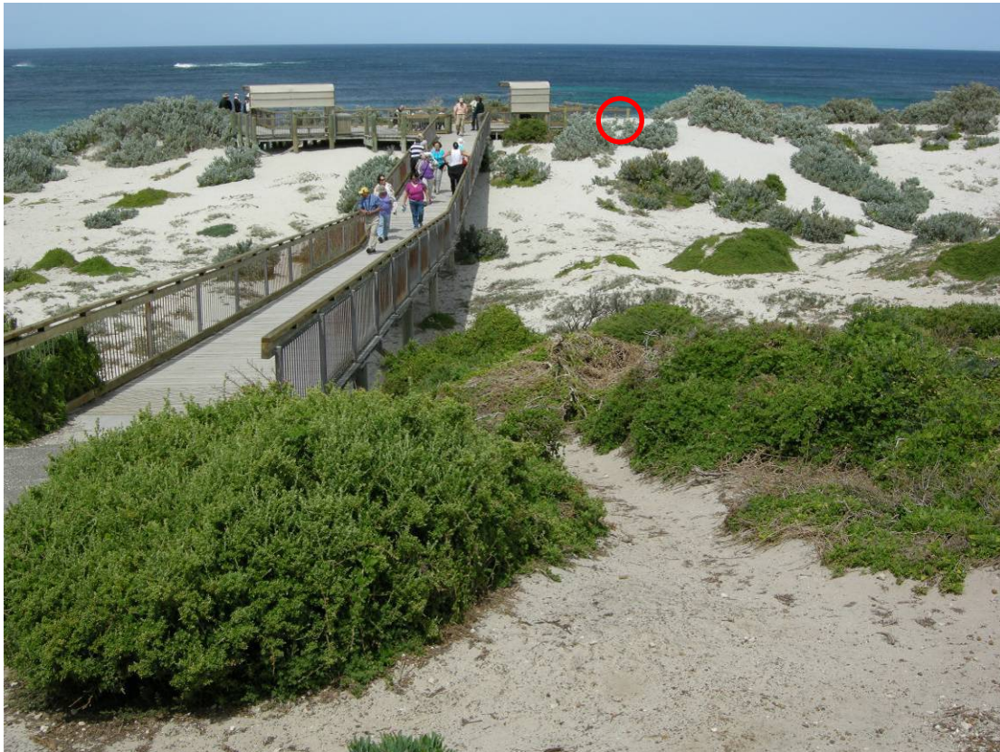
Fig. 9. View to South just off the asphalt section of the path from the Visitor Centre to the Main Platform. The new bridge will commence from where the photographer is located and will extend to the north-western corner of the Main Platform (circled). The new bridge would be wider and approximately 700mm higher than the current bridge. The pier footings supporting the bridge can also be seen in the picture—these footings would be replaced and the number would be increased, particularly where the bridge is to be widened.
