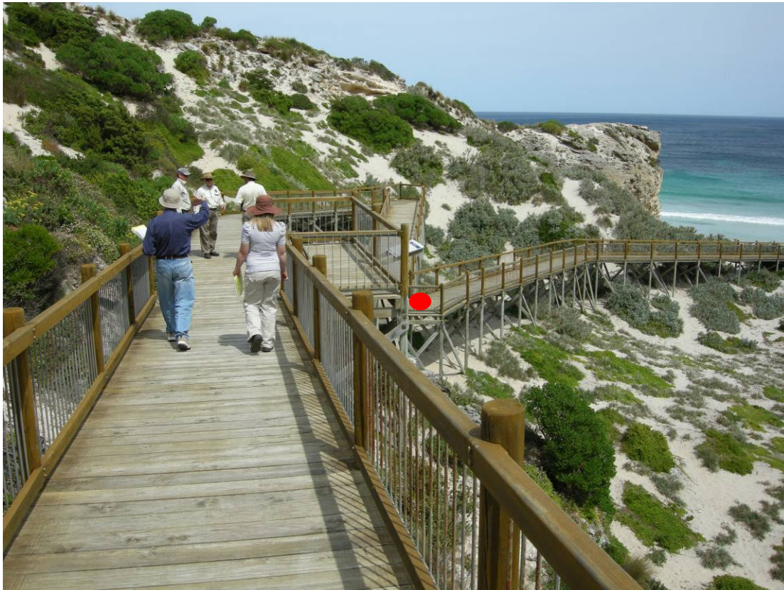
Fig. 20. View to the South taken from between turn two and turn three on the Don Dixon Boardwalk. Near the centre of the picture is a red dot, which indicates the location of turn four, which may be widened to accommodate more tourist interpretation facilities.
