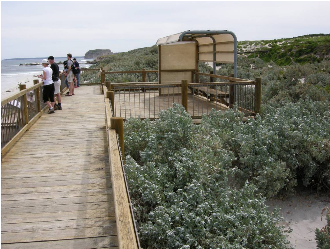
Fig. 21. View to the West taken on the platform at the end of the Don Dixon Boardwalk. This platform may be widened (into the dunes, not the beach).
