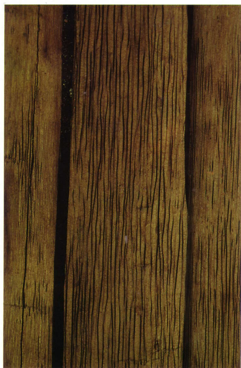
10. Upper. Roof corners are held in position with hollowed-out trunks of Veitchia macdanielsii , Olpoi village, west Espiritu Santo. 11. Lower left. Detail of house wall constructed of split trunks of Veitchia macdanielsii ; the black sclerotic fibers within the cortex of the trunk make an attractive pattern (Lakatoro, Malakula). 12. Lower right. Roadside food stall bench constructed of split trunks of Veitchia macdanielsii (Wormet, Malakula).
