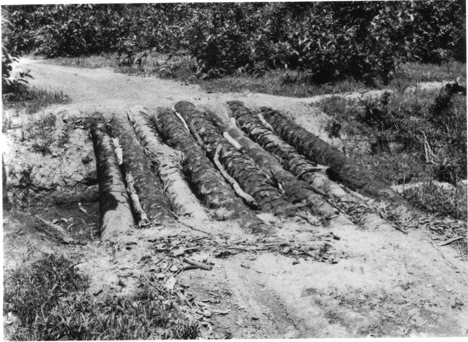
7. Oil palm trunks used for bridge construction near Jabicunda.
