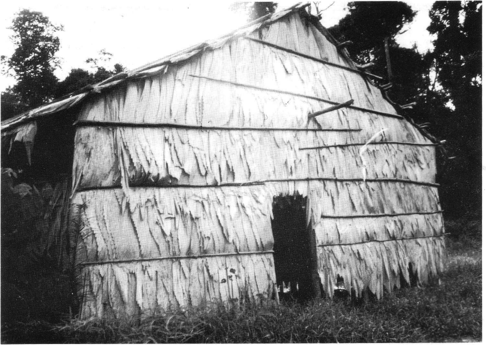
2. Rain will not penetrate or leak through any shelter properly thatched with "Joey's" leaves.
