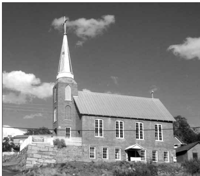
The restored St. Augustine's Cultural Center, Austin, Nevada. The new roof, repaired windows, walls, steeple, and dry stack foundation are readily seen. The small building to the right of the picture (unrestored) was the office of Dr. William W. Wixom, a local physician. He was the father of Emma Wixom (1859–1940), who went on from local music training to become a famous international operatic singer, adopting the stage name “Emma Nevada.” The family is said to have attended St. Augustine's. Photo: Michael D. Friesen
