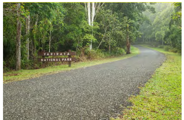
Figure 37: Entrance to VNP, 2017
