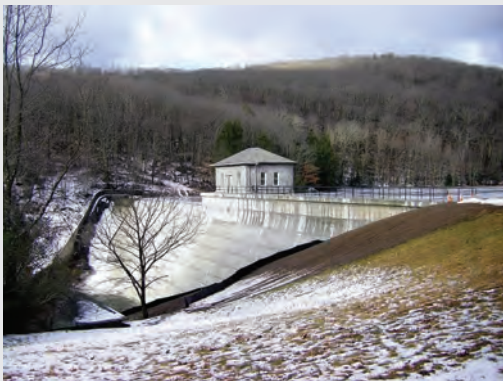
Upper Shepaug Dam Photo Warrenhistoricalsociety.org
