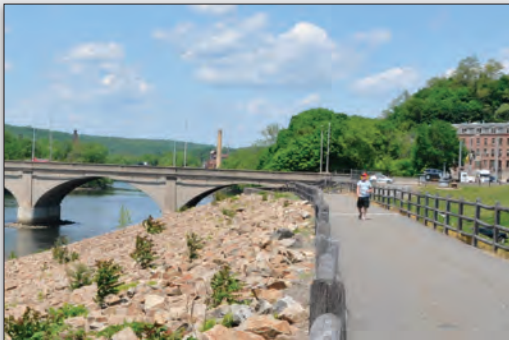
Section of Local Flood Protection Project. Photo: NVCOG
