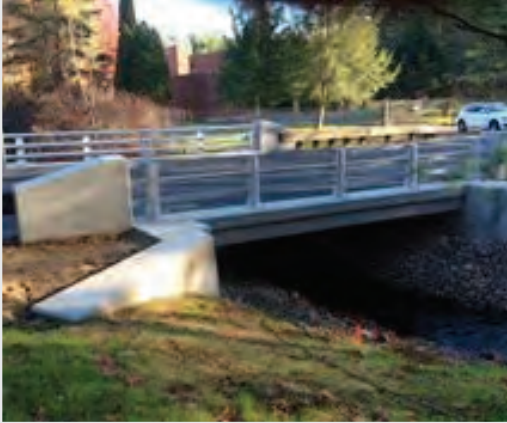
The new Blacks Road Bridge Photo CheshireCT.org
