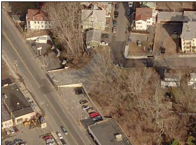
Figure 3-10: Repaired Landslide Site at Southview Street and South Main Street, Waterbury
