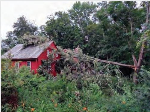
Tree damage from Isaias in Woodbury Photo: Jennifer O'Brien
