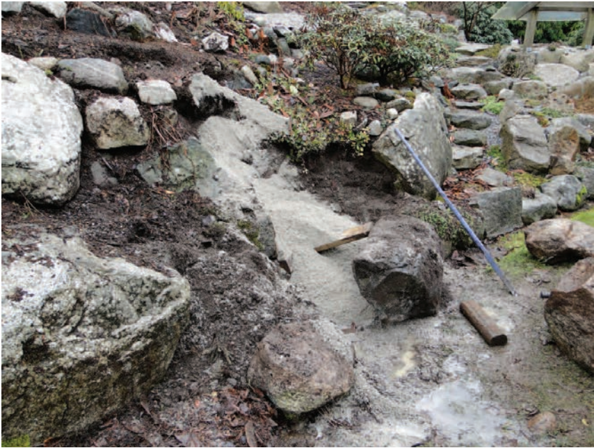
Backfilling the foundation rock with coarse sand
