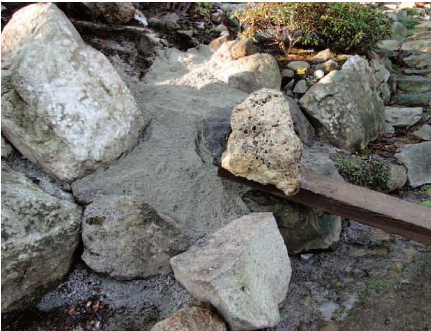
Sliding a piece of tufa into place
