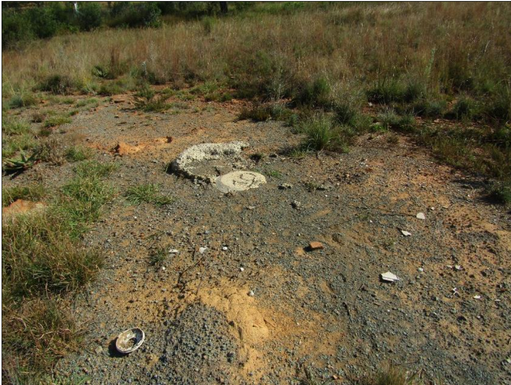
FIGURE 18: BOREHOLE TEST PIT REHABILITATION REQUIRED
