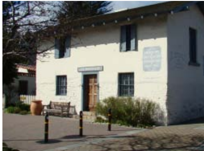
Protect adobe materials from deterioration.
