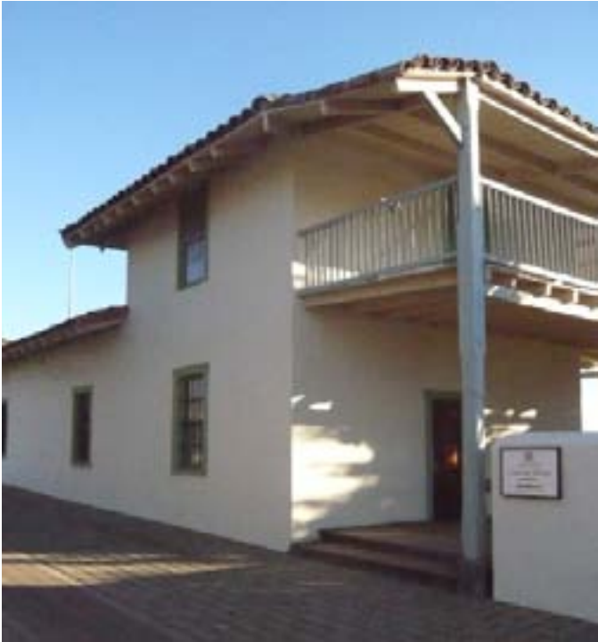
Roof forms are varied, although gable and hip roofs are predominant. Note the clipped roof form on the Custom House.
