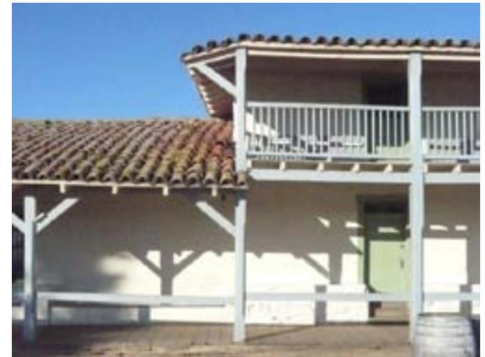
Preserve original roof materials.
