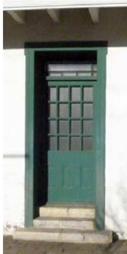
Maintain the original proportions of a historically significant door.
