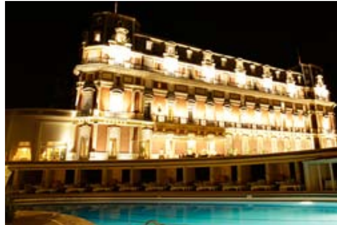
Discouraged: Building wall lighting too bright and not well shielded.
