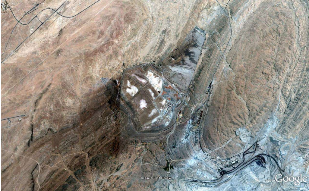
Figure 3.12: Location and lay-out of the tailings facility at Rössing
