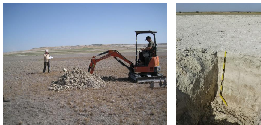
Figure 5. All soil profiles for description and sampling purposes were dug with a backhoe machine.
