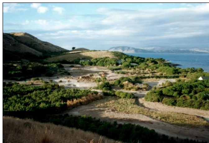
Figure 47. Before the Water The “Waikoko Wetland” construction prior to flooding with water.
