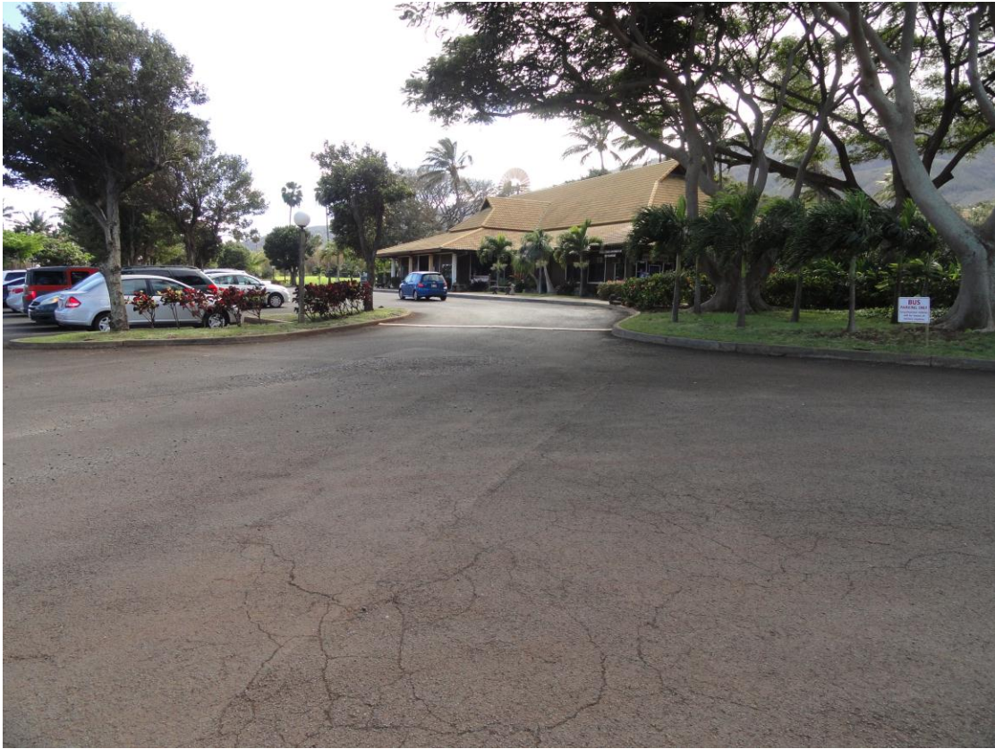
Figure 2 – Entrance to the Maui Tropical Plantation facilities
