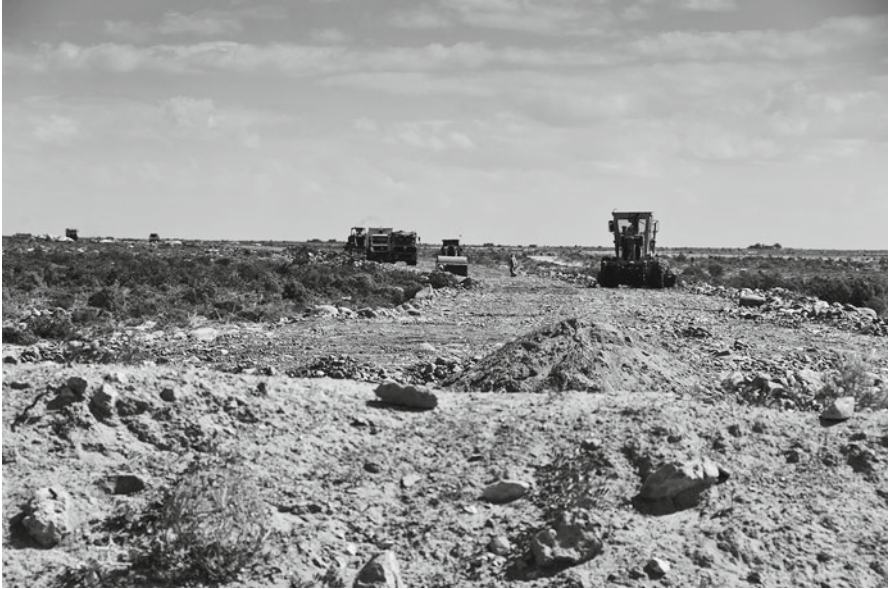
Fig. 7.20 Construction of a new road on the Naged plain. December 2008
