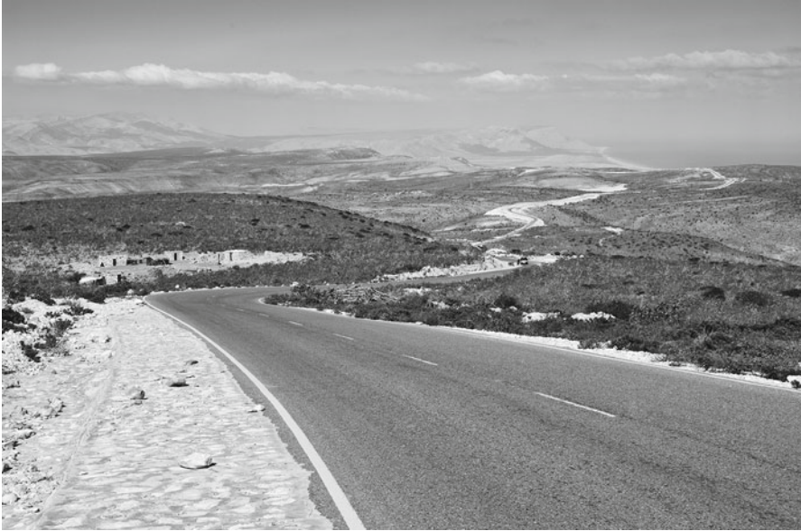
Fig. 7.22 The new Dixam road links the north and south of the island. December 2008
