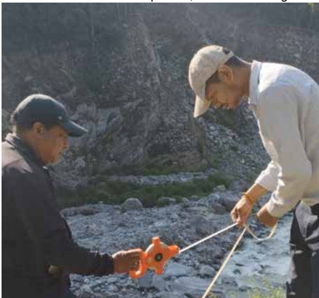
Measurement of amount of sand and boulders deposited at Melamchi river
