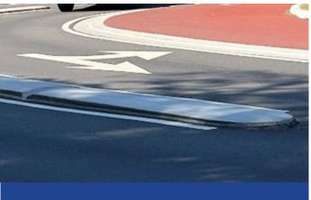
FIGURE 3. RAISED PAVEMENT CHARACTERISTICS OF TURBO ROUNDABOUT. SOURCE: FHWA
