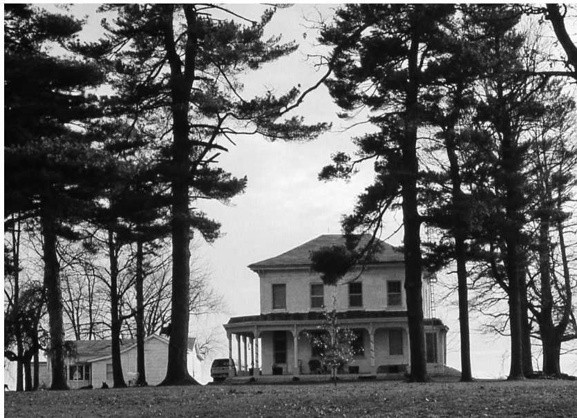
Figure 3. The home built by Elihu Hall south of Athens, Illinois.
