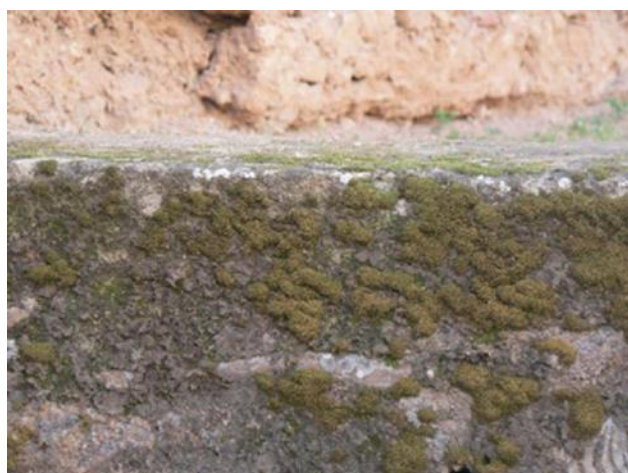
Fig.10: Vertical edge of the calcarenite basin of ablution in Chellah covered by bryophytes
