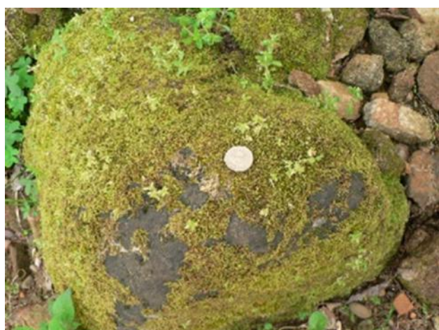
Fig.11: Total recovery by bryophytes of an architectonic element and loss of legibility
