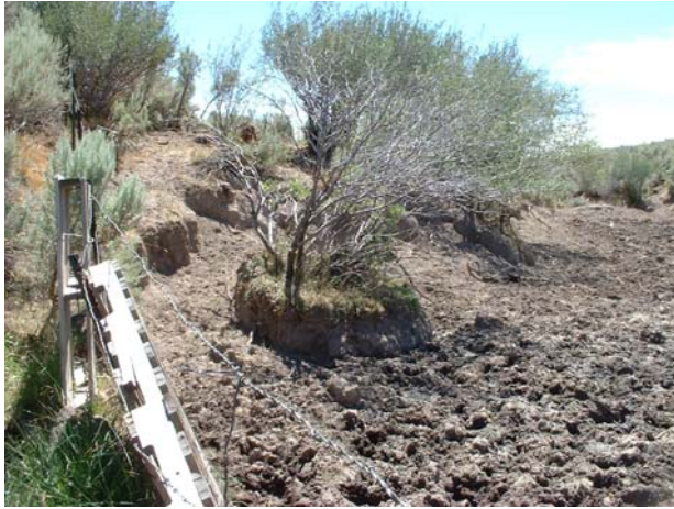
Figure 3. Rock Creek. Just s of fence at s border of Lonigan Springs. Facing se.
