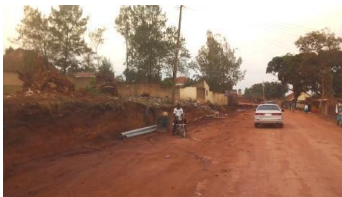
Source: Last Mile ESIA Field Photo
