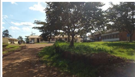
Part of the Mukono DLG offices to be connected Source: Last Mile ESIA Field Photos 2017
