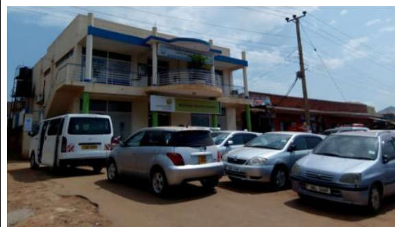
National Water and Sewerage Corporation, Kitintale Source: Last Mile ESIA Field Photos 2017
