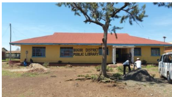
Bugiri District Public Library Source: Last Mile ESIA Field Photos 2017
