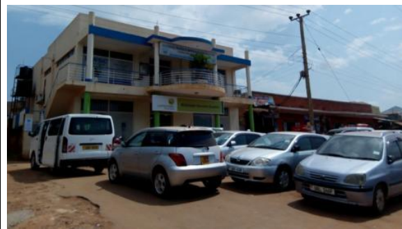
National Water and Sewerage Corporation, Kitintale Source: Last Mile ESIA Field Photos 2017
