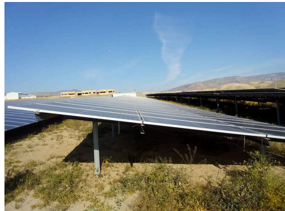
Footpaths laid out for cleaning and maintenance purposes in Deir Alla PV wheeling farm, which is a similar project that the SEED project previously delivered to Deir Alla Municipality, Jordan Valley
