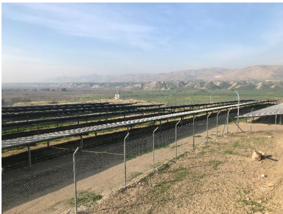
Footpaths laid out for cleaning and maintenance purposes in Deir Alla PV wheeling farm, which is a similar project that the SEED project previously delivered to Deir Alla Municipality, Jordan Valley
