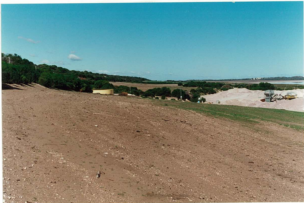
View looking South - East over mined out areas to east of the plant buildings and feed stockpiles. Areas in the foreground and middle distance have recently had the topsoil replaced.
