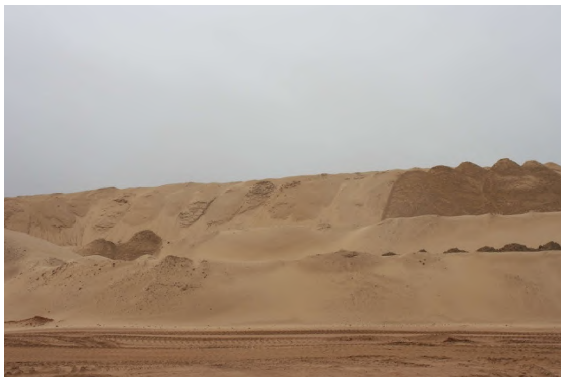
Plate 1 Mine Pit Undergoing Backfilling (Hose Mine)
