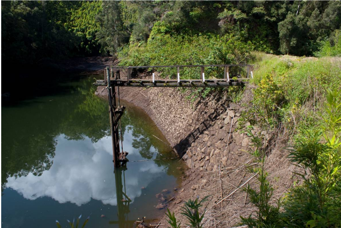
Figure 1-3. View of the Existing Reservoir and Catwalk
