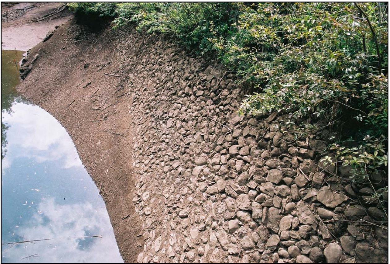
Figure 16. Feature D, the dam view to south.
