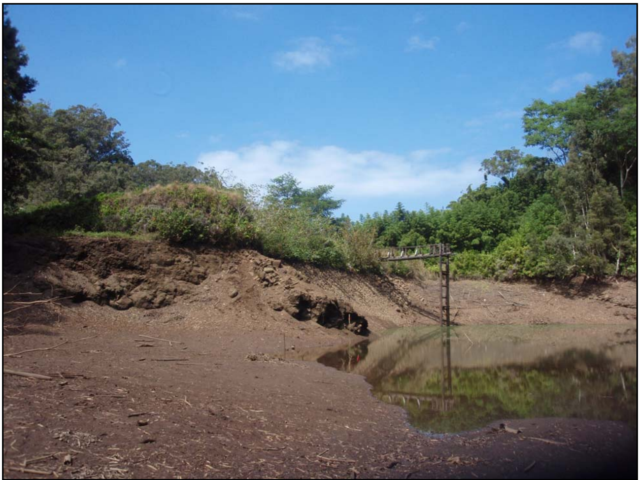
Figure 4. Overview of the Kolea Reservoir, view to north.
