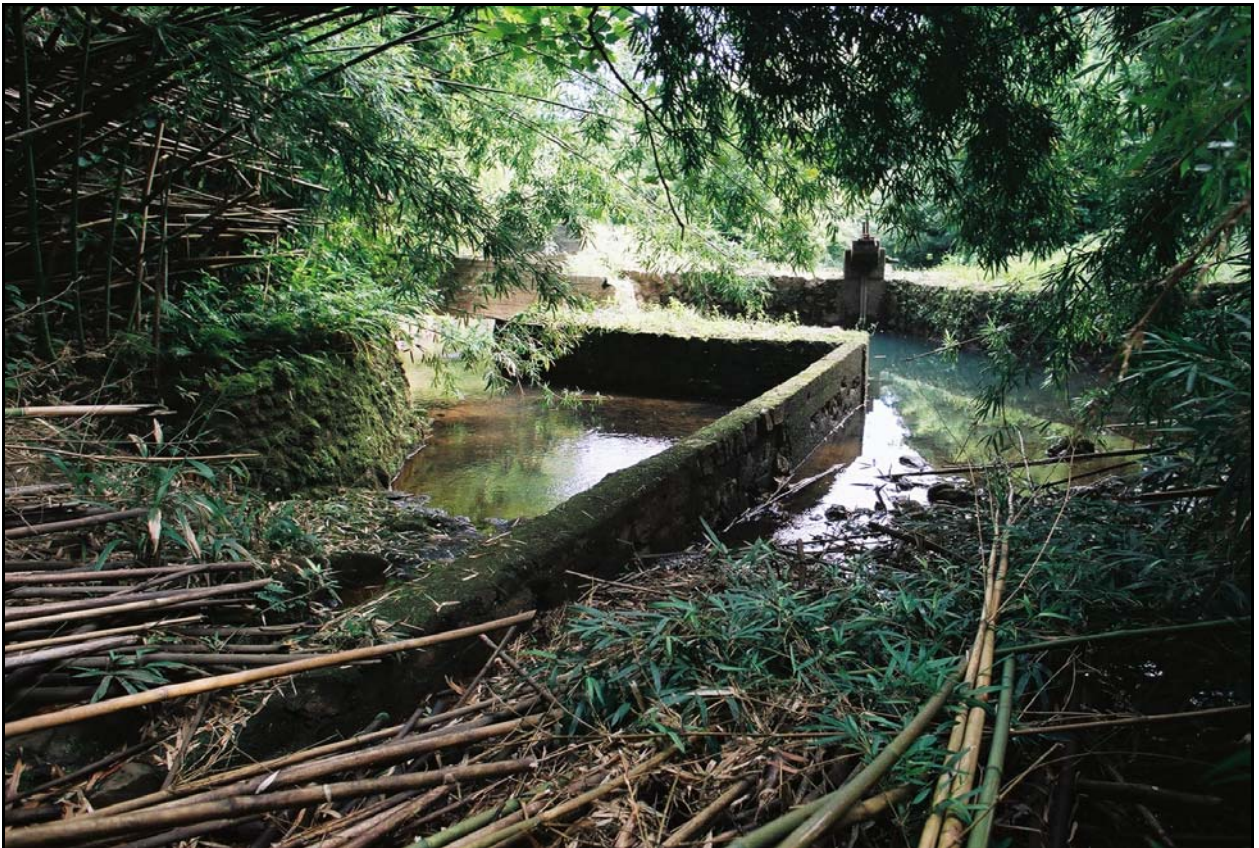
Figure 18. Feature F, the water diversion controls, view north.
