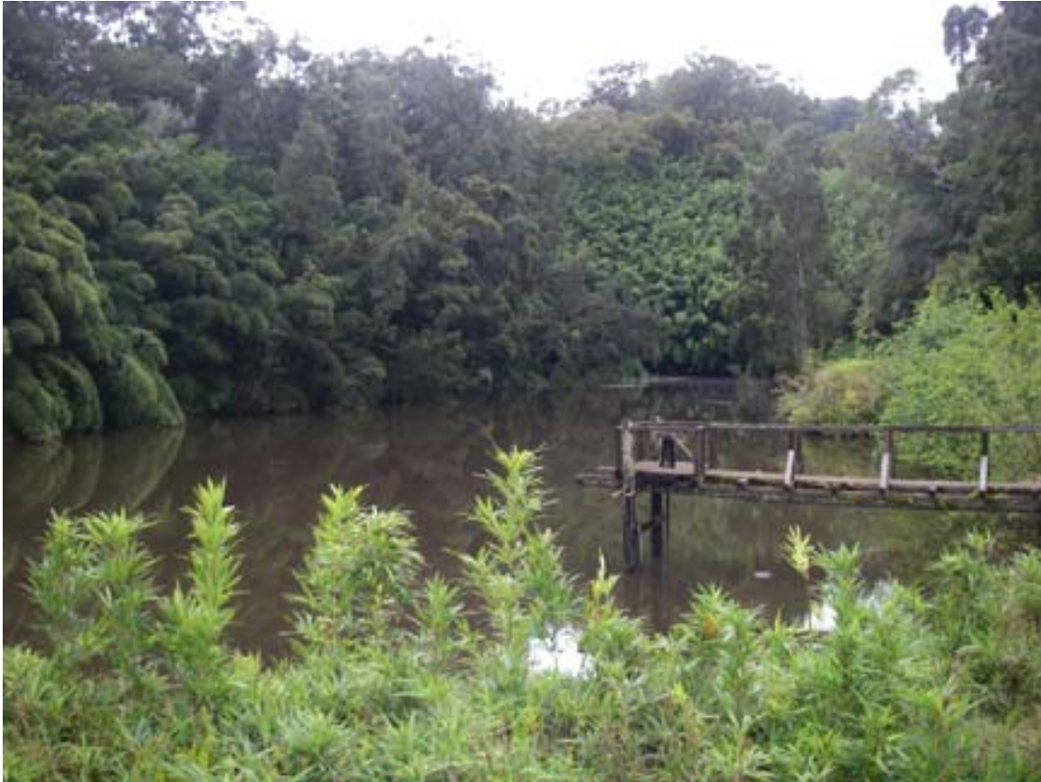
Figure 2. Kōlea Reservoir looking upstream from the north end of the dam.
