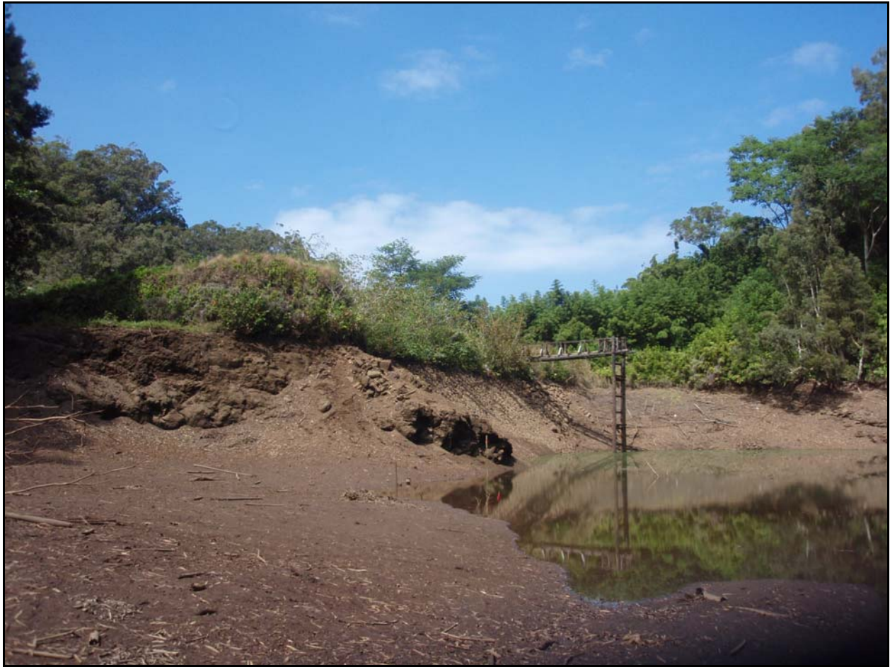
Figure 3. Overview of the Kolea Reservoir, view north.
