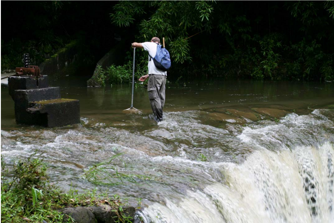
Figure 5. Kōlea Stream at Manuel Luis Ditch at a time of above normal flow. In this photo, the ditch flows from left to right just beyond the biologist's net. Kōlea Stream flows in from background left and, at high flow, over the approximately 18-ft (6-m) dam in the foreground right. The valve at left allows diversion of water via a pipe to the stream bed downstream of the dam structure.
