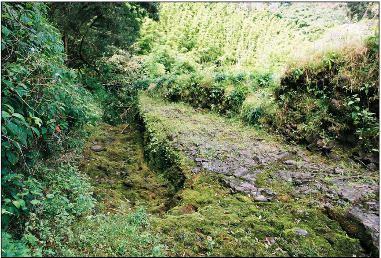
Figure 14. Feature A, spillway, view to west.
