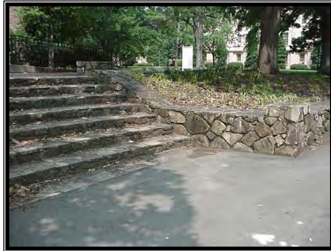
Chatham Stone wall and Steps at Memorial Hall
