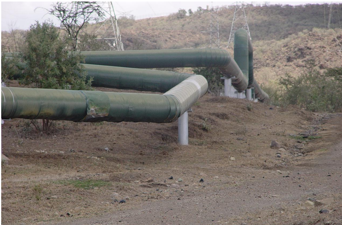
Figure 2.8: The plant and pipelines painted to a color that camouflages with the surrounding environment.
