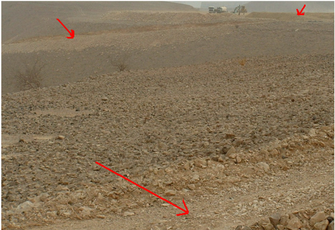
Plate 7.9a. Roads created by oil working activities have resulted in compaction of the soil surface (red arrow).
